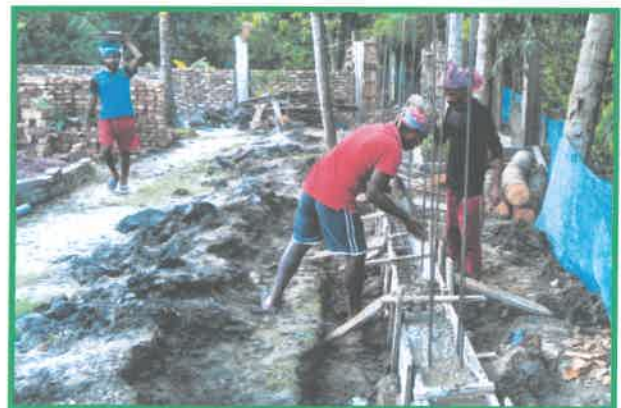
Construction of Khulna Church wall
